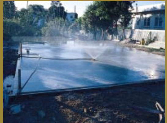
Figure 9: Curing concrete using a sprinkler
