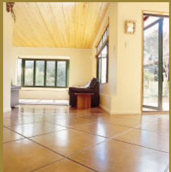
A coloured concrete floor with cut joints
