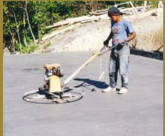
Figure 8: Power floating
